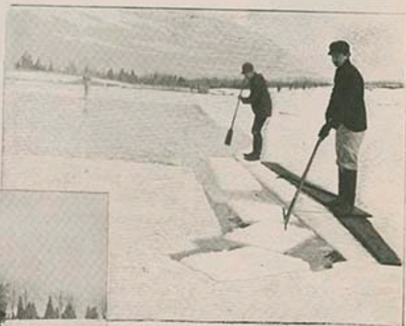
Breaking Loose and Floating the Cakes of Ice
