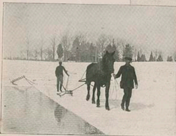
Plowing the Ice—One of the Cutting Processes
