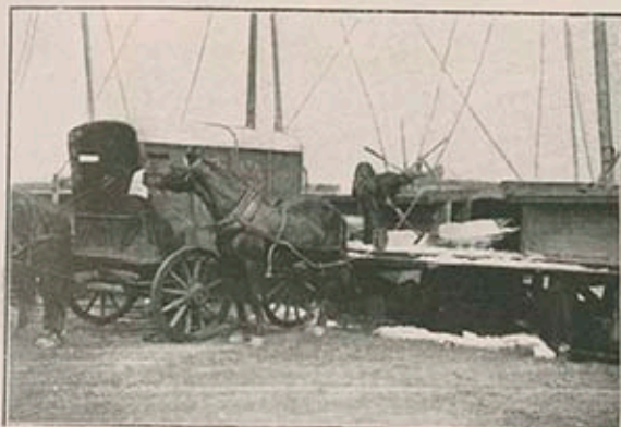
Unloading Ice at the Dock
