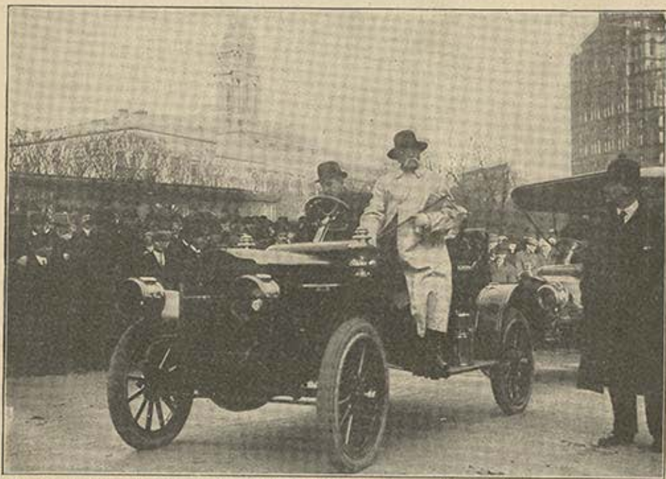
Weston alighting from an automobile at City Hall Square, New York City. To the right is seen the "World" Building—the City Hall is the white structure in the background.
