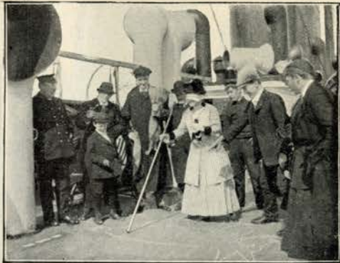
Photo No. 2.—Placing the Pig's Eye
