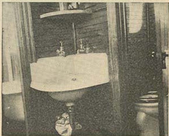
Showing how separate compartments have been made of bathroom and toilet, with the wash basin in the hall at the entrance of each.
