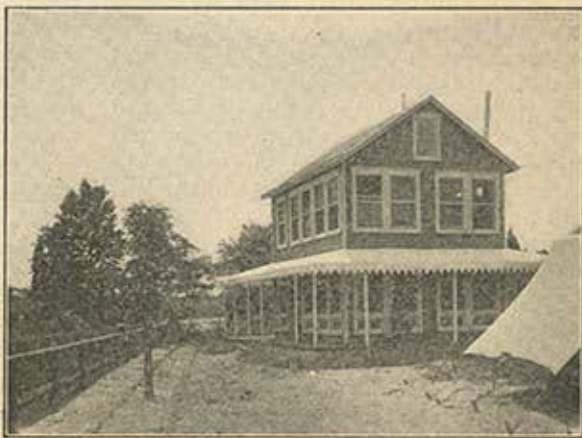
Showing Position of the House and Yard.—Instead of being built in line with the fence, as is usual, the position of the house has been so arranged, that the sunlight comes into every window at some hour of the day.
