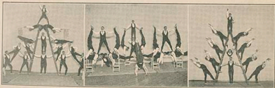
There is Almost no Limit to the Variety of Effects That Can be Produced Through the Building of These Specimens of "Human Architecture"
