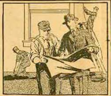
Be an Electrical CONTRACTOR
