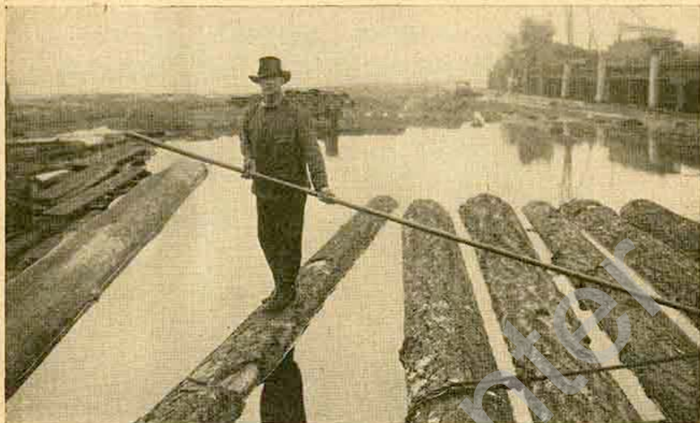
This kind of work requires dexterity.
