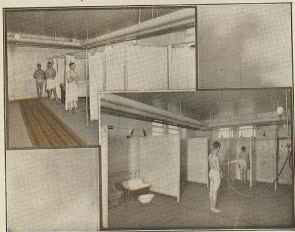
Two sections of the Men's Water-Treatment Department.
