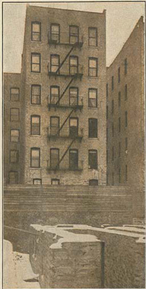
This photograph of the rear of a "flat-house" shows the unsatisfactory provisions for light and air even of the "new law" tenements. Lower floors, in rear, are hopelessly dark and poorly aired. When the foreground is built up similarly, the buildings, back to back, will have only a narrow space between, as indicated at the right of the picture.
